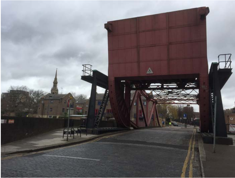
One of the many drawbridges over the waters, leading to wharfs
